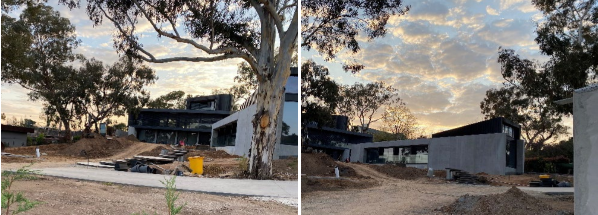
Figure 1: New residence constructed in Deakin.
