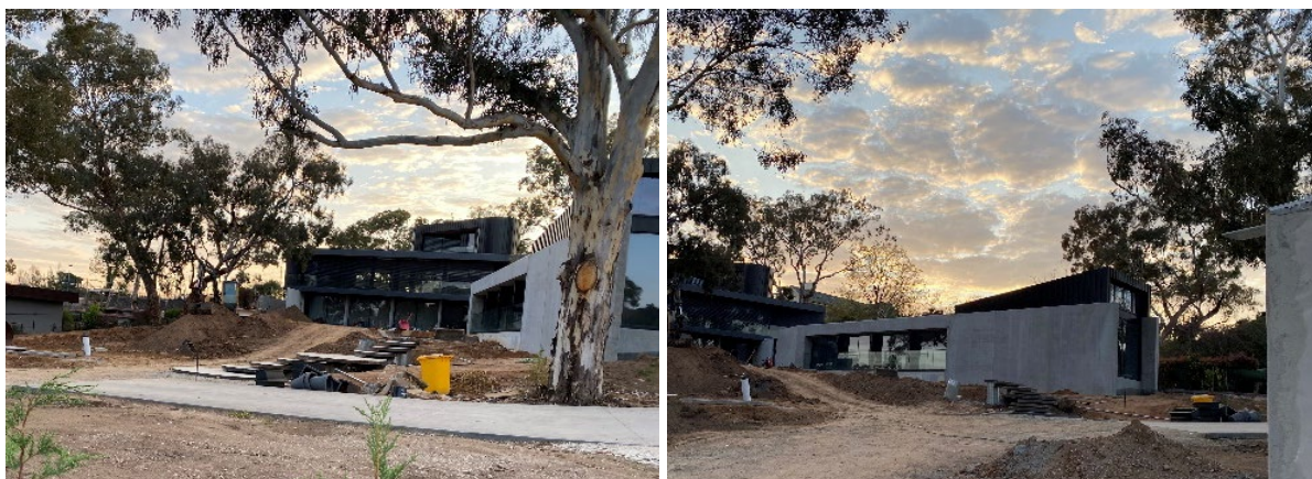
Figure 1: New residence constructed in Deakin.
